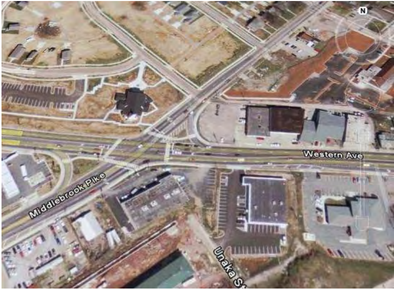
Figure 3-30 Western Avenue near Middlebrook Pike
