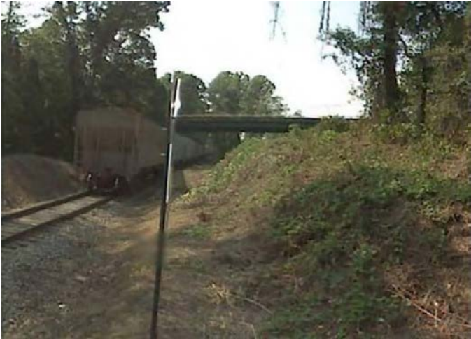
Figure 3-82 Overpass at SR 168
