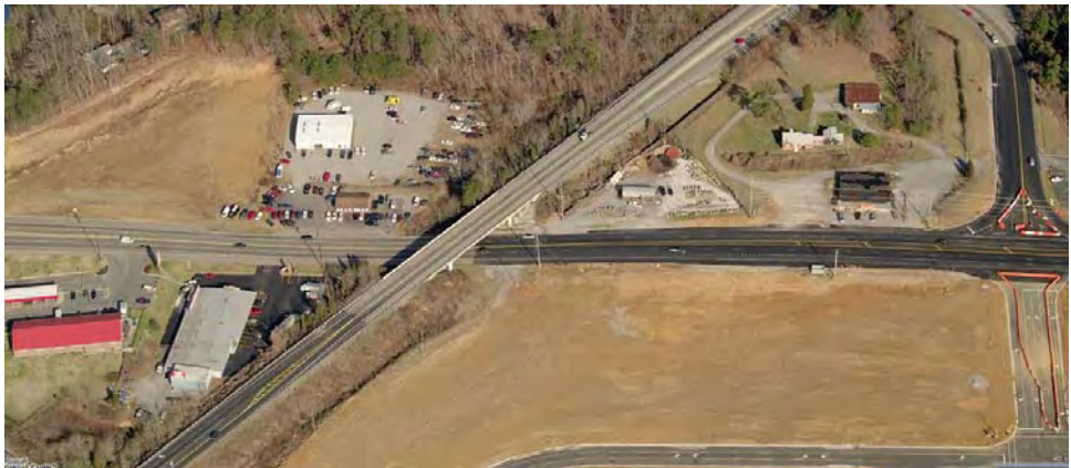
Figure 3-73 Sevier Highway Passing over Chapman Highway
