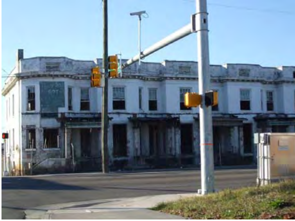
Figure 3-43 Dilapidated Building on North Broadway near Rescue Mission
