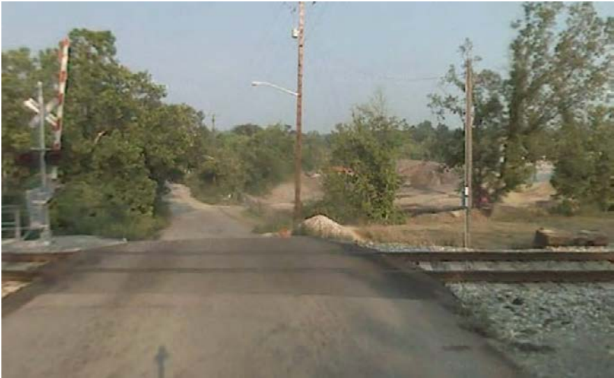
Figure 3-80 Rail Crossing at Candora Road
