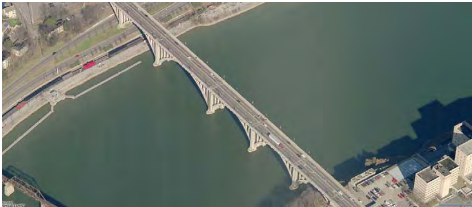
Figure 3-70 Traffic on Henley Street Bridge
