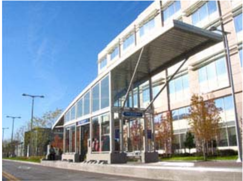
Cleveland Euclid Corridor Bus Rapid Transit Station
