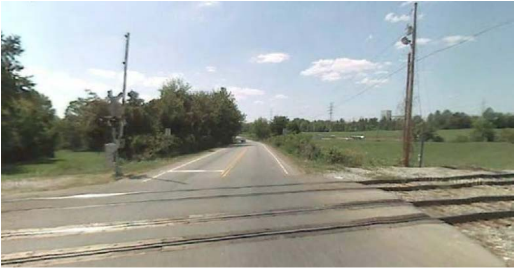
Figure 3-83 Double Tracks near Alcoa Plant
