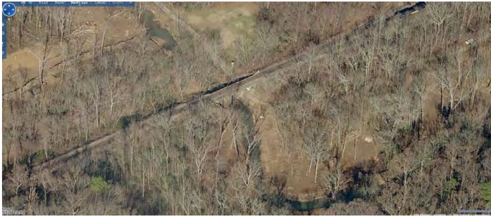
Figure 3-19 Bridge over Third Creek
