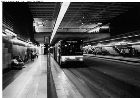
Figure 2-6 Seattle Busway Tunnel
