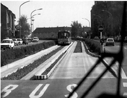
Figure 2-5 Guided Bus, Essen, Germany
